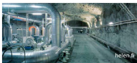
Energy tunnel in Helsinki
